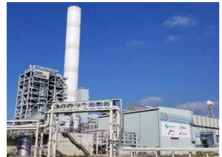
Osaki CoolGen facility, Japan.
