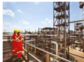
Above: Petra Nova Carbon Capture, United States of America; right: Quest Facility, Canada. Photo courtesy of Shell.
